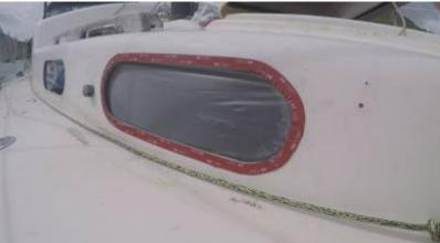
This is the tricky part. The method I used was to pull the red protective film on the VHB tape just enough that I had a tab I could pull from between the window and the tape. I then placed the window
