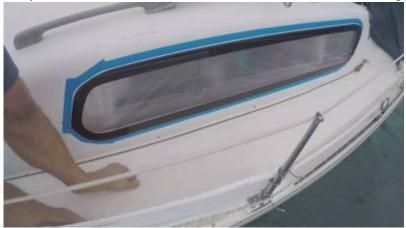
I used Dow-Corning 795 sealant, which is also structural. To make sure I filled the gap between the window and hull, I used a syringe.
