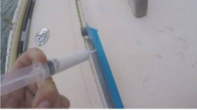
Make sure you remove the masking tape before the sealant cures, and preferably immediately after application.
